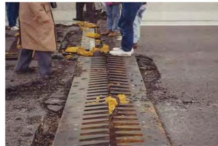
Photo 1 Damage of the expansion joint
